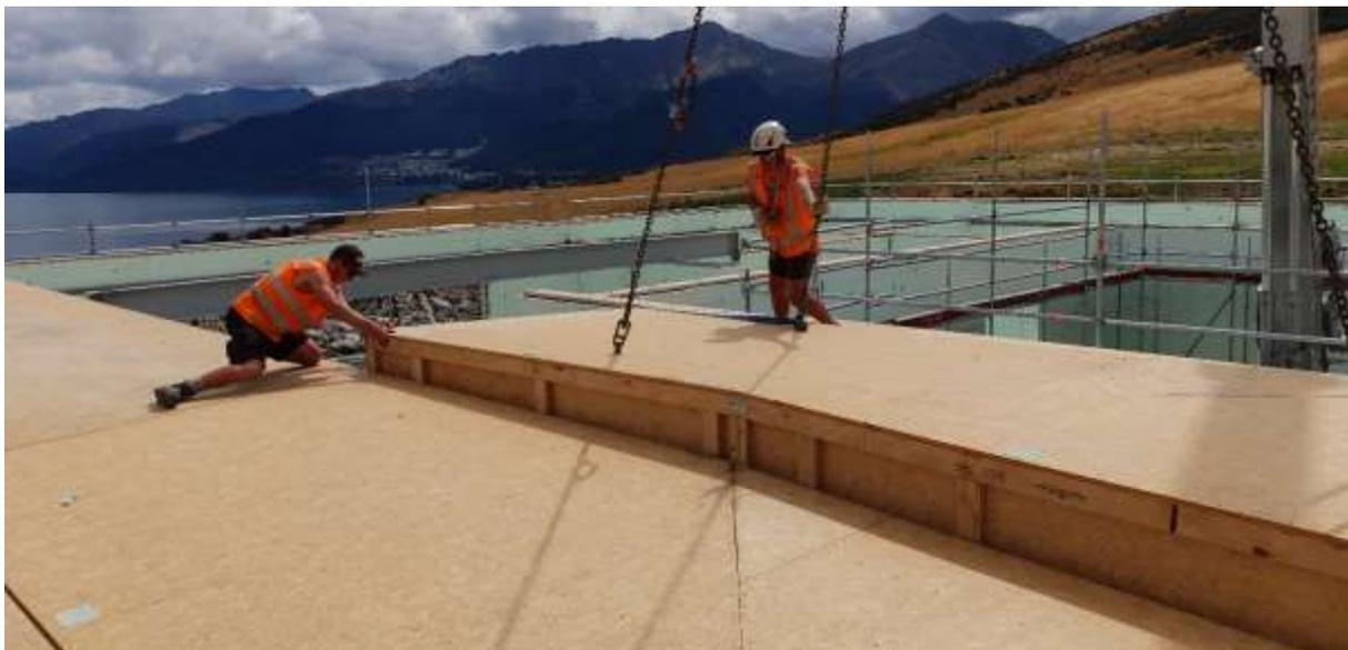
*Figure 4: Lifting in a residential midfloor using lifting hooks (Wasp)*
