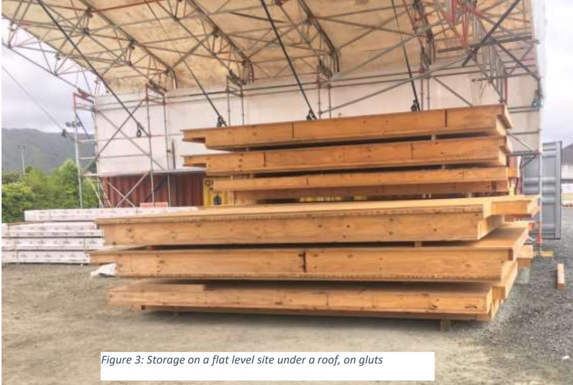
*Figure 3: Storage on a flat level site under a roof, on gluts*
