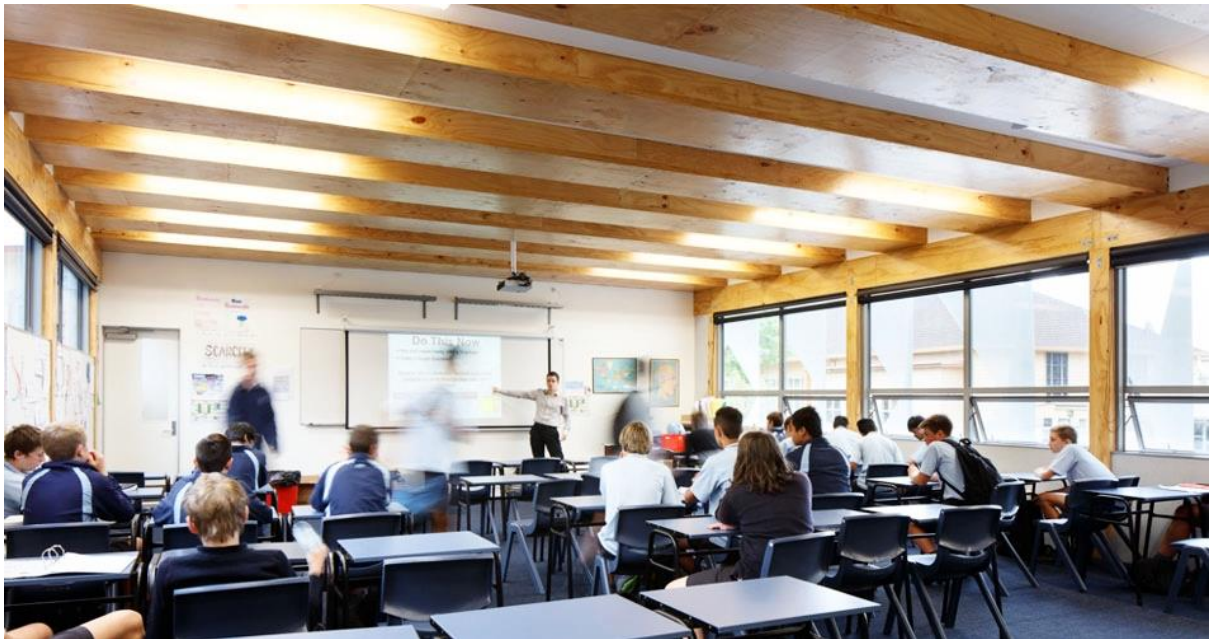
Figure 1: Nelson College - A two storey classroom teaching block with a Potius midfloor.
