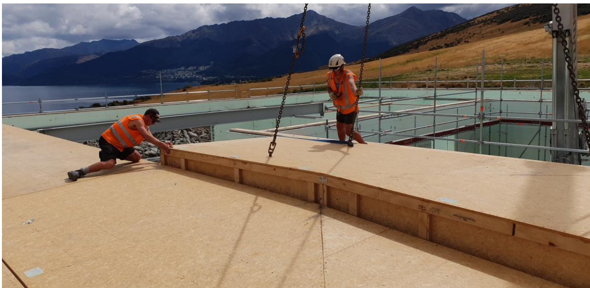
Figure 4: Lifting in a residential midfloor using lifting hooks (Wasp)
